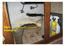
There is a leak on the hot water shut-off valve below the sink, which should be repaired
